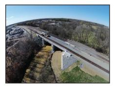
The proposed bridge was a 160-foot-long, threespan structure, located adjacent to an existing railroad bridge. Once construction began, Crowder realized the bridge design was virtually impossible to construct. Carrying more than 30 trains per day, the existing bridge had to remain in service during construction. It became apparent that the proposed high-wall abutment foundations would be in direct conflict with the existing bridge foundations.
