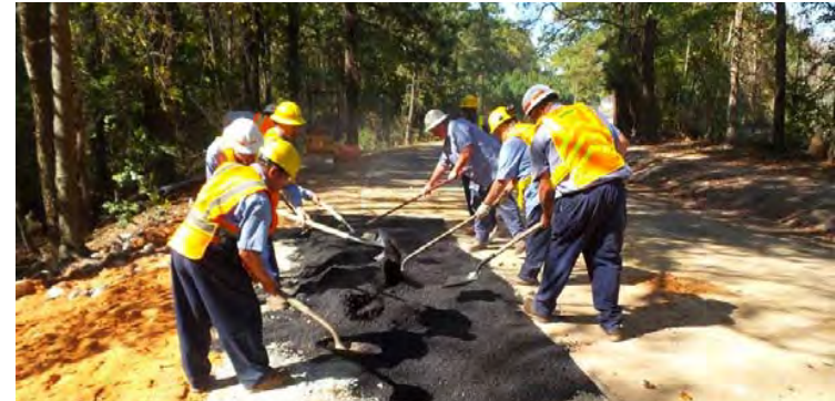
Shoulder and lane repairs
