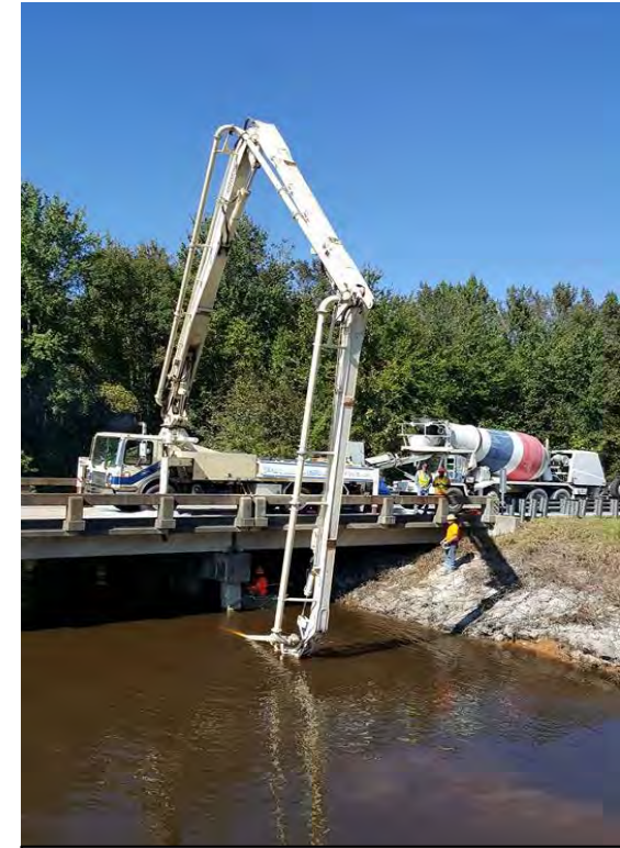
I-95 Bridge Foundation Repairs
