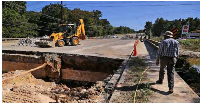
Monticello Road Bridge End Repairs
