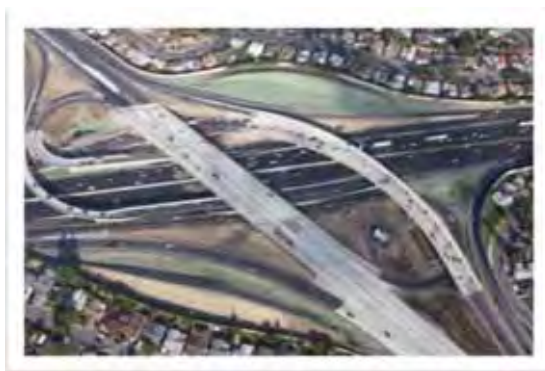
Reconstruction of I-880/SR92 interchange
