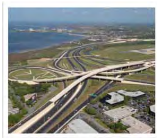
SR60 Tampa Airport/Interchanges
