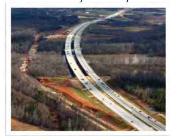
I-85/Yadkin River Bridge Salisbury, NC
