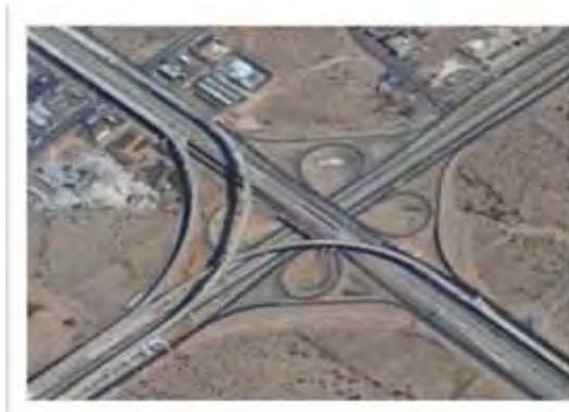
Loop 375 at I-10 Interchange
