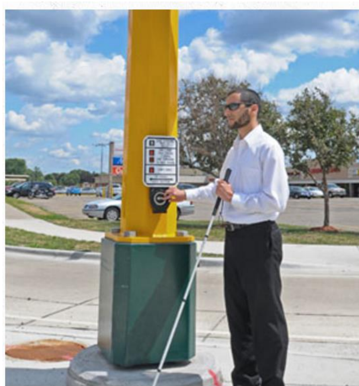
Accessible Pedestrian Signals (APS)
