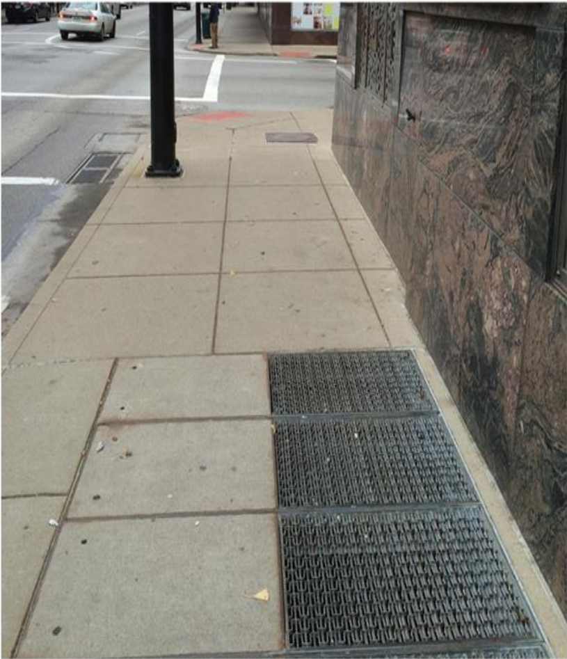
/R303.3.3 — shall not be located on curb ramps, blended transitions, landings, or gutters within the PAR/
